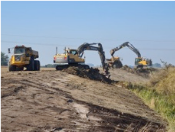
Digging activity, phase 2. Photo Johnny Carlsson
