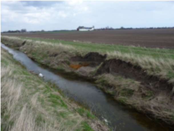
View of the Tullstorpsån stream area at Sånarp before the wetland construction. Soil erosion is contributing to the sediment content in the water. Photo: Johnny Carlsson
