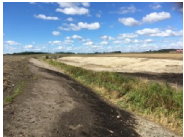
A two-step ditch at Sillesjö. Photo Ingrid Stjernquist
